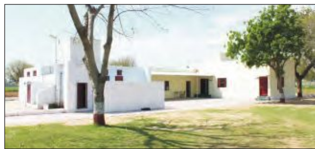
The newly renovated staff quarters for the Manager & Dairy workers along with one Guest room were formally made operational in the month of January 2015.
