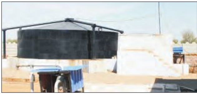
To make full use of Cow dung, a 60 metric ton Capacity Bio-Gas (Gobar Gas) Plant was installed & commissioned at Smt. Urmila Chaudhary Dairy Farm, Bahal in the month of February 2015.
